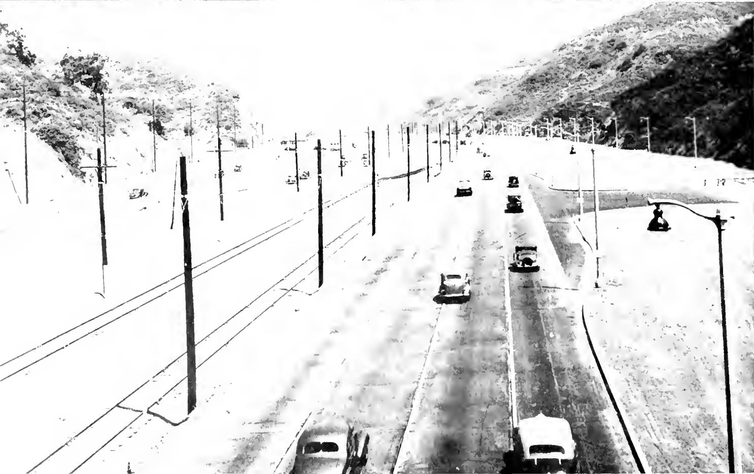
Views of two sections of Caluenga Pass Freeway in Los Angeles County that was reconstructed into a 12-lane divided highway largely with gas tax funds totaling $886,000. Additional funds were contributed by PWA, Los Angeles City and County
